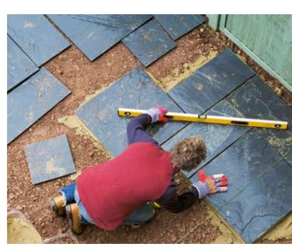
You need to leave a 1cm (1/2 in) gap between each slab, which you'll fill in later with mortar. As you progress, use your spirit level or a plank of wood to ensure the slabs are level with the pegs you banged into the ground earlier.
