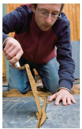
Fill the gaps between the paving slabs using a pointing trowel and the same mortar mix as you used before. Try not to get mortar on the slab surfaces, as again this will stain if it's allowed to set.
